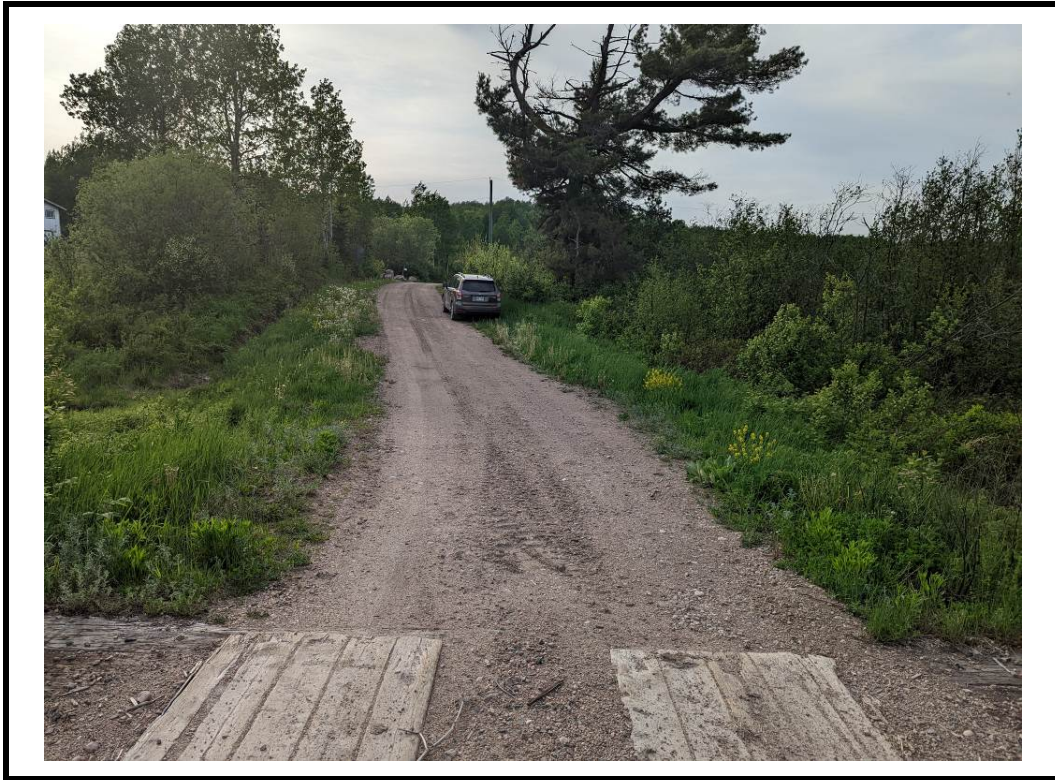
Photo 3 North approach from centre of structure
