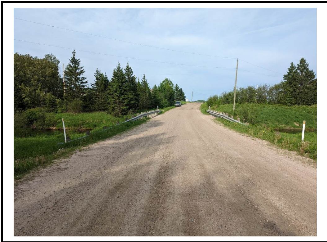
Photo 2 Structure from west approach
