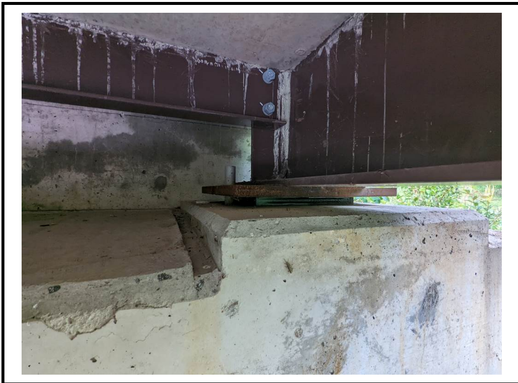
Photo 12 Typical bearing at southeast corner
