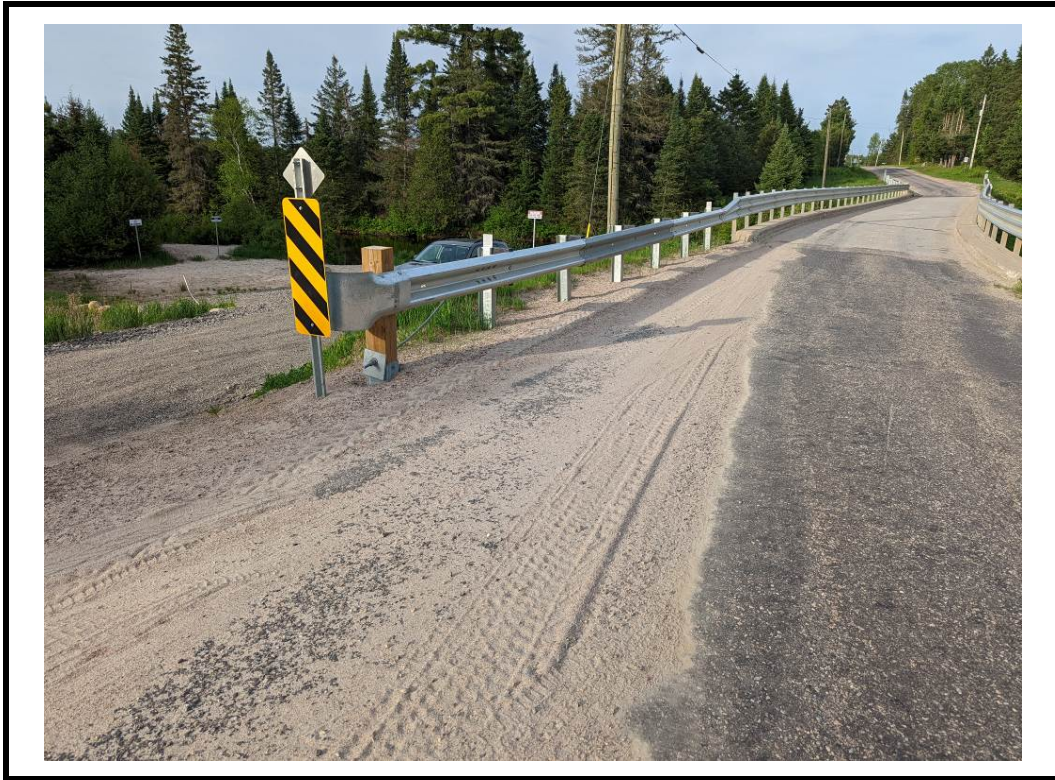
Photo 7 Typical approach barrier at northwest corner
