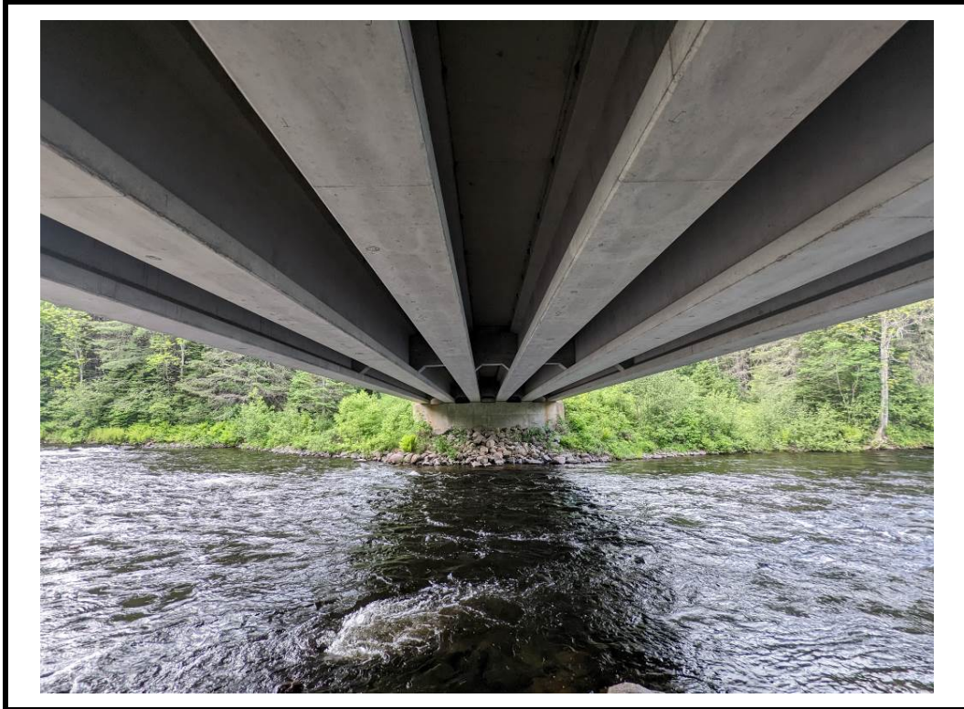
Photo 11 Underside of Structure
