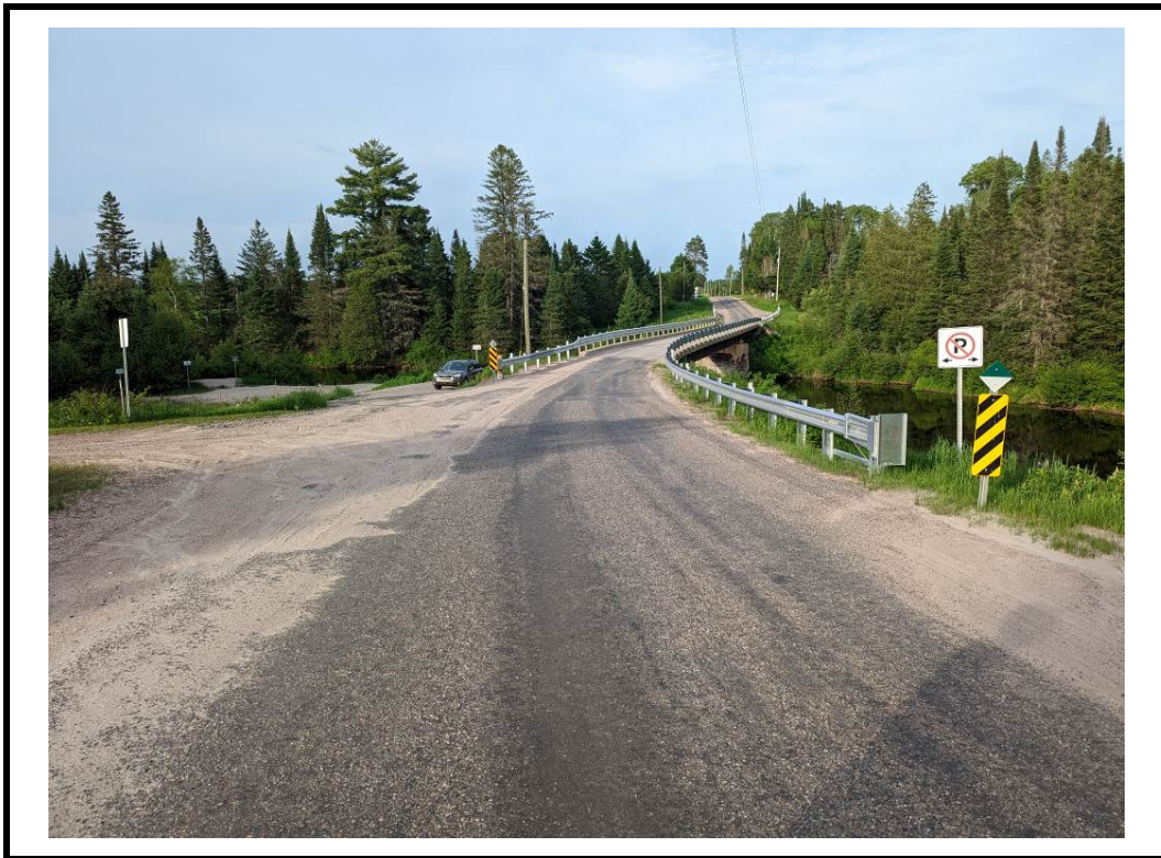
Photo 2 Structure from west approach
