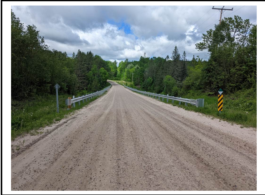
Photo 1 Structure from east approach
