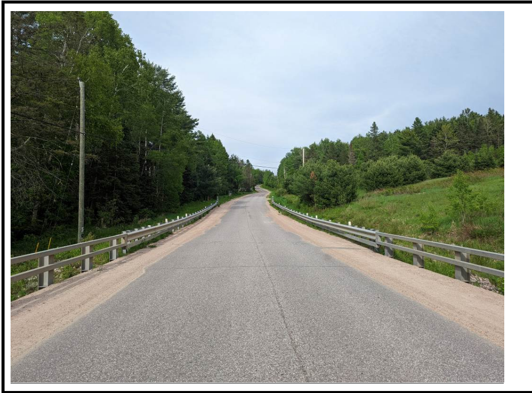
Photo 3 East approach from centre of structure
