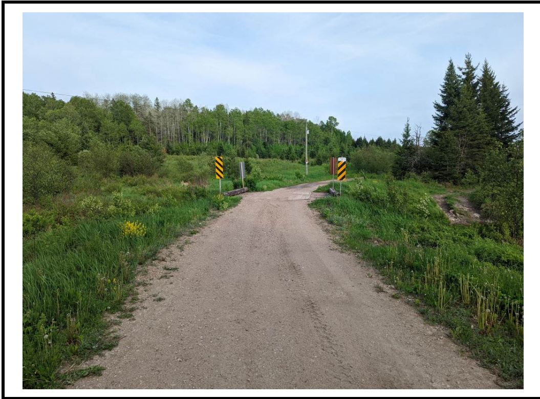
Photo 1 Structure from north approach
