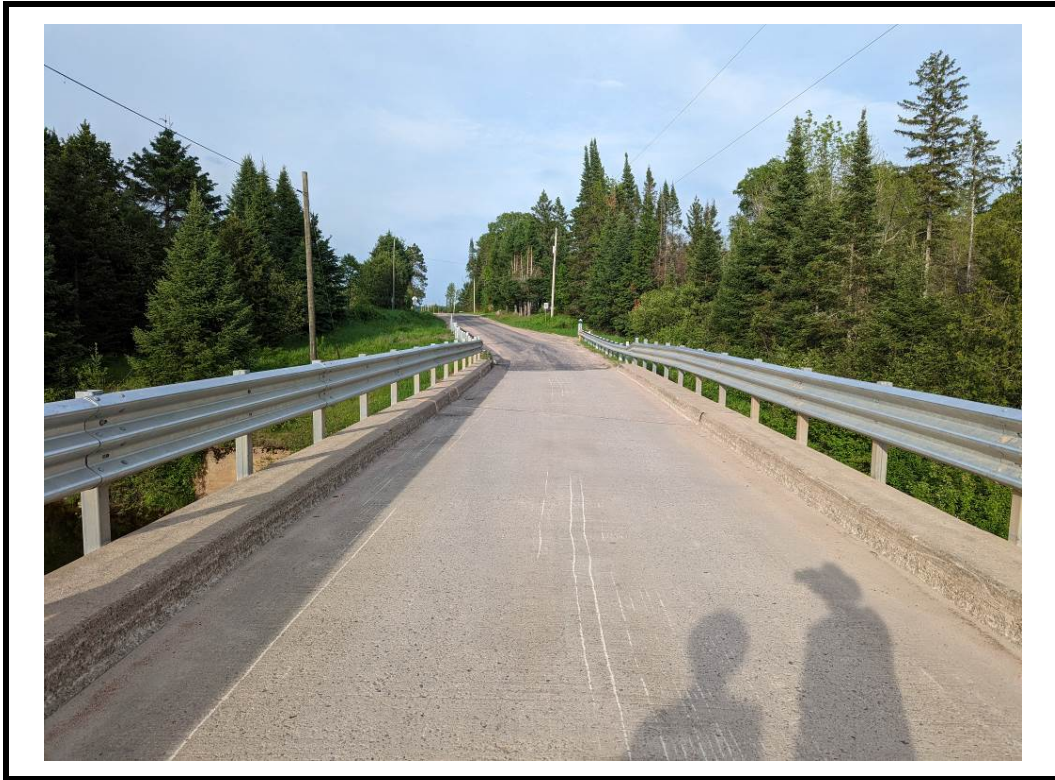
Photo 3 East approach from centre of structure
