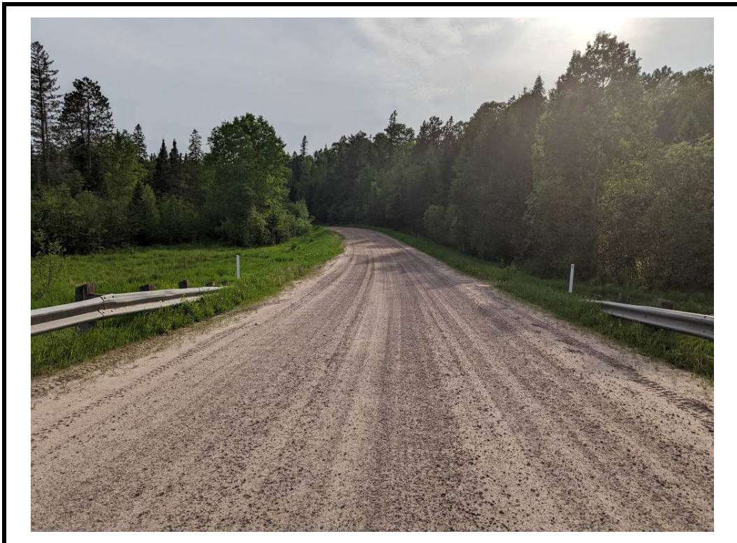
Photo 4 West approach from centre of structure
