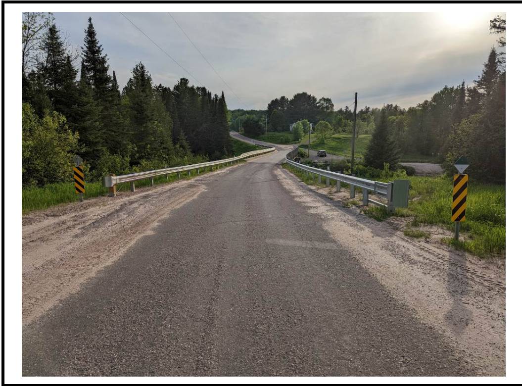
Photo 1 Structure from east approach
