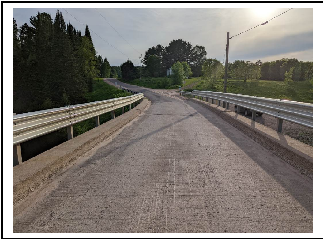
Photo 4 West approach from centre of structure
