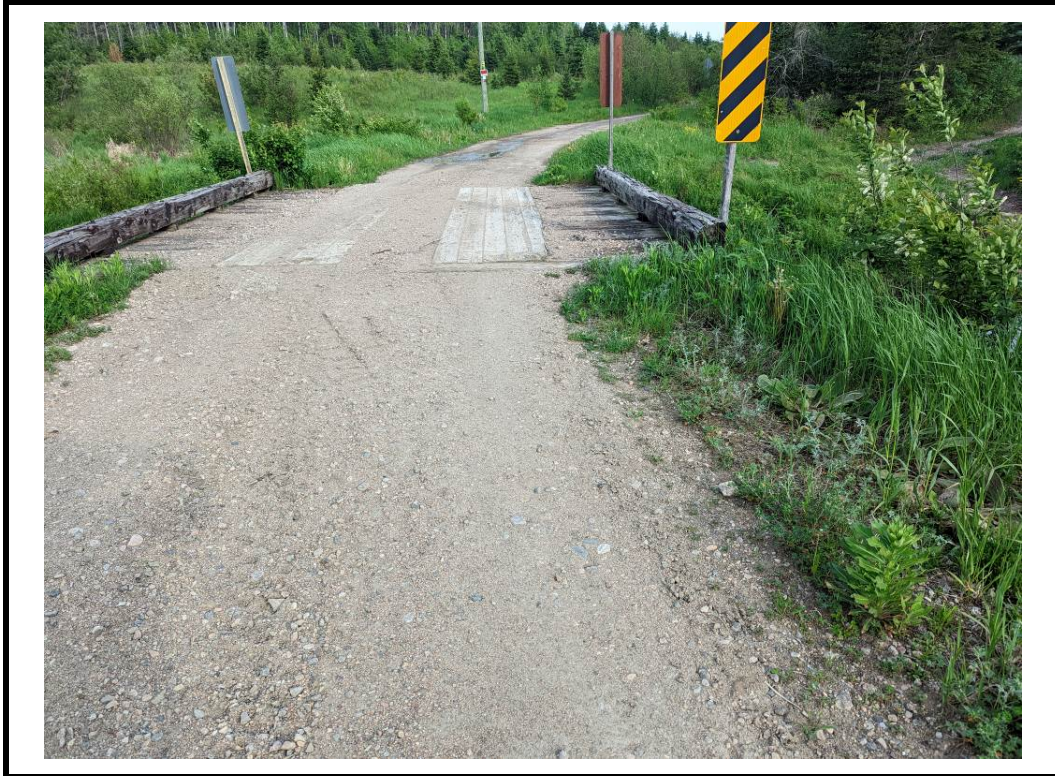
Photo 7 Damaged hazard sign on NW corner of barrier
