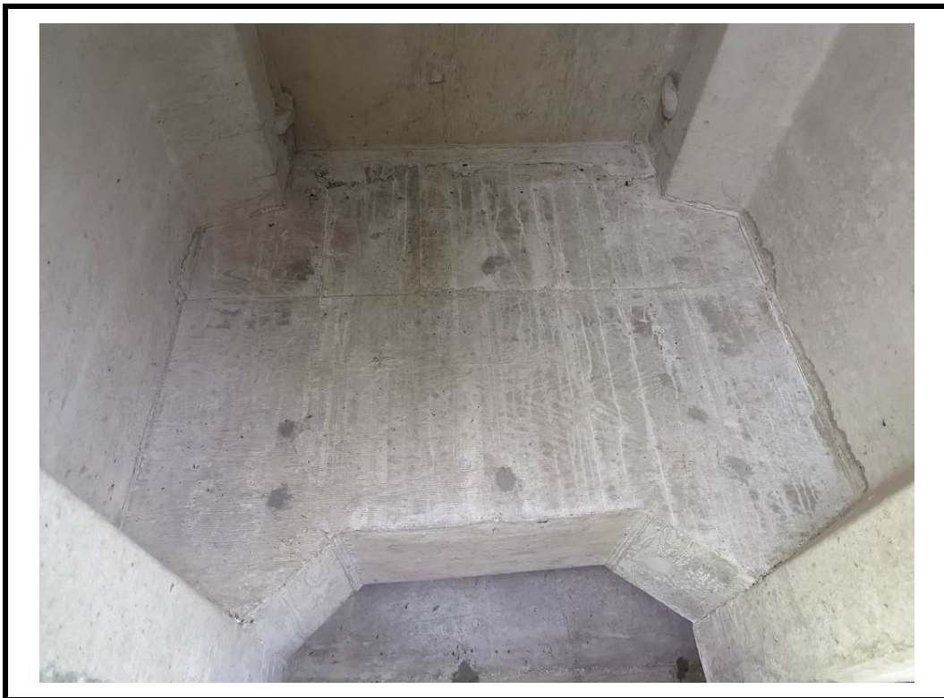
Photo 16 Typical view of diaphragm at west
