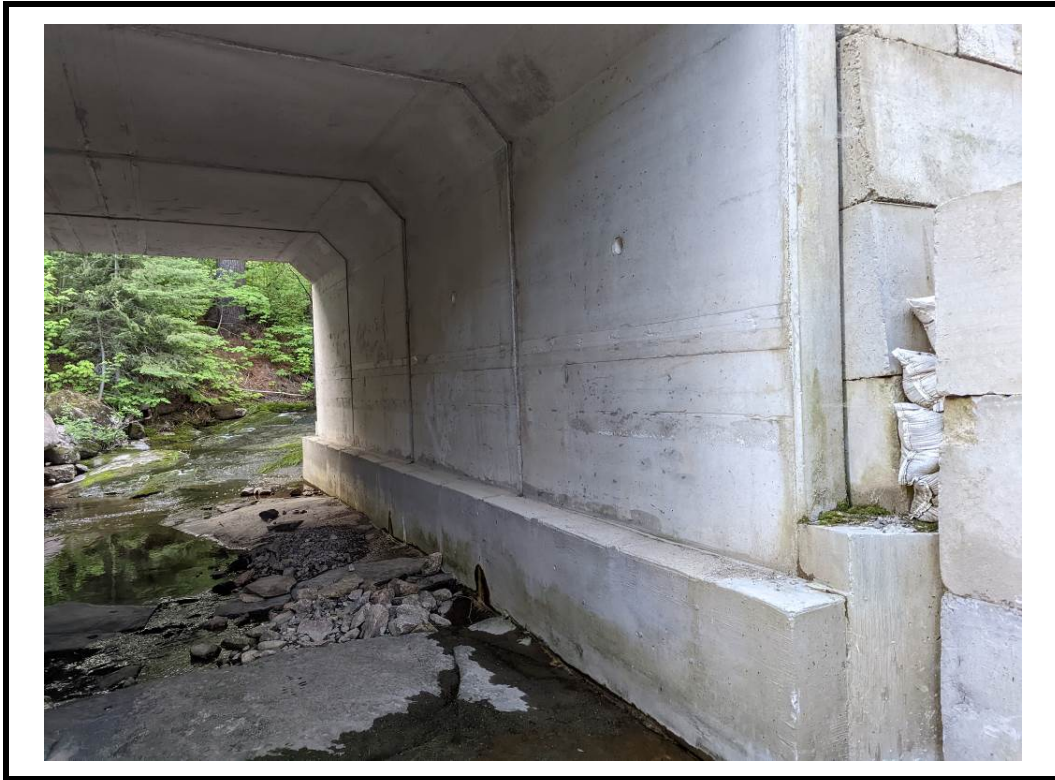
Photo 13 West abutment wall
