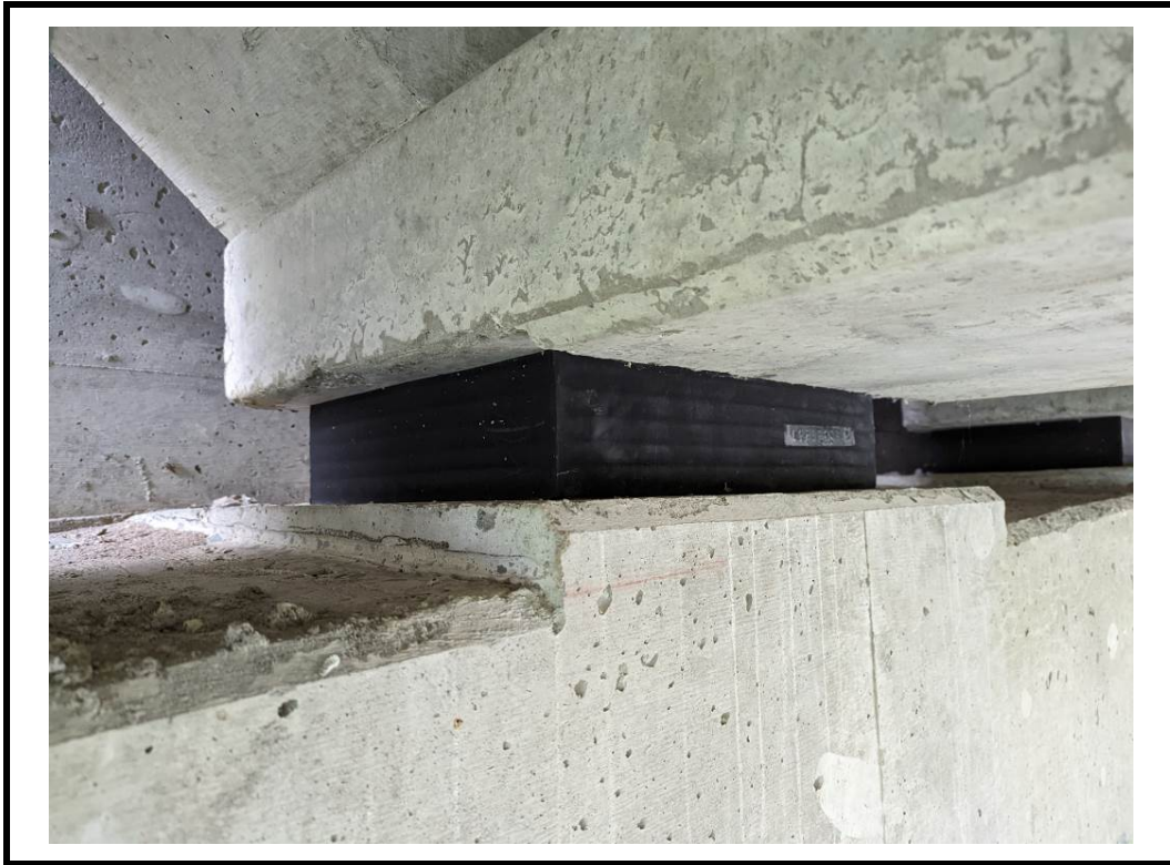
Photo 15 Typical bearing at east abutment wall
