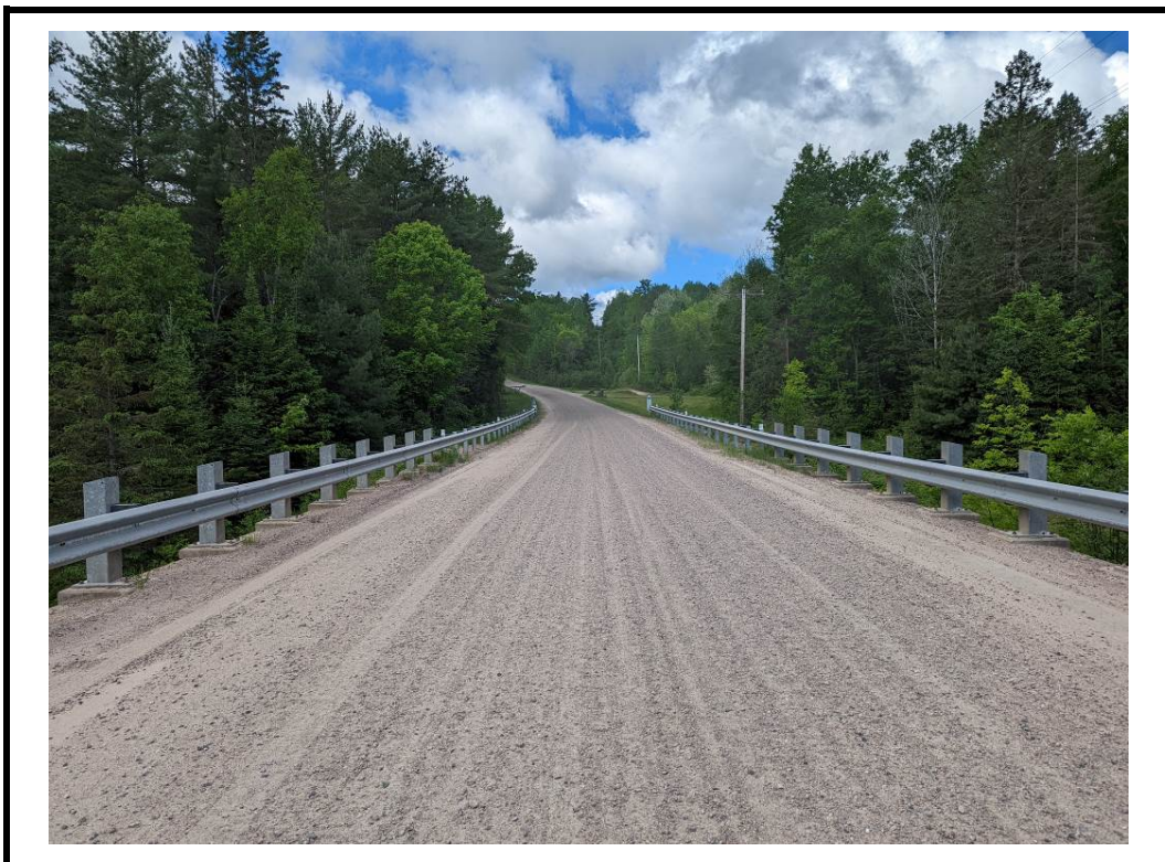
Photo 4 West approach from centre of structure
