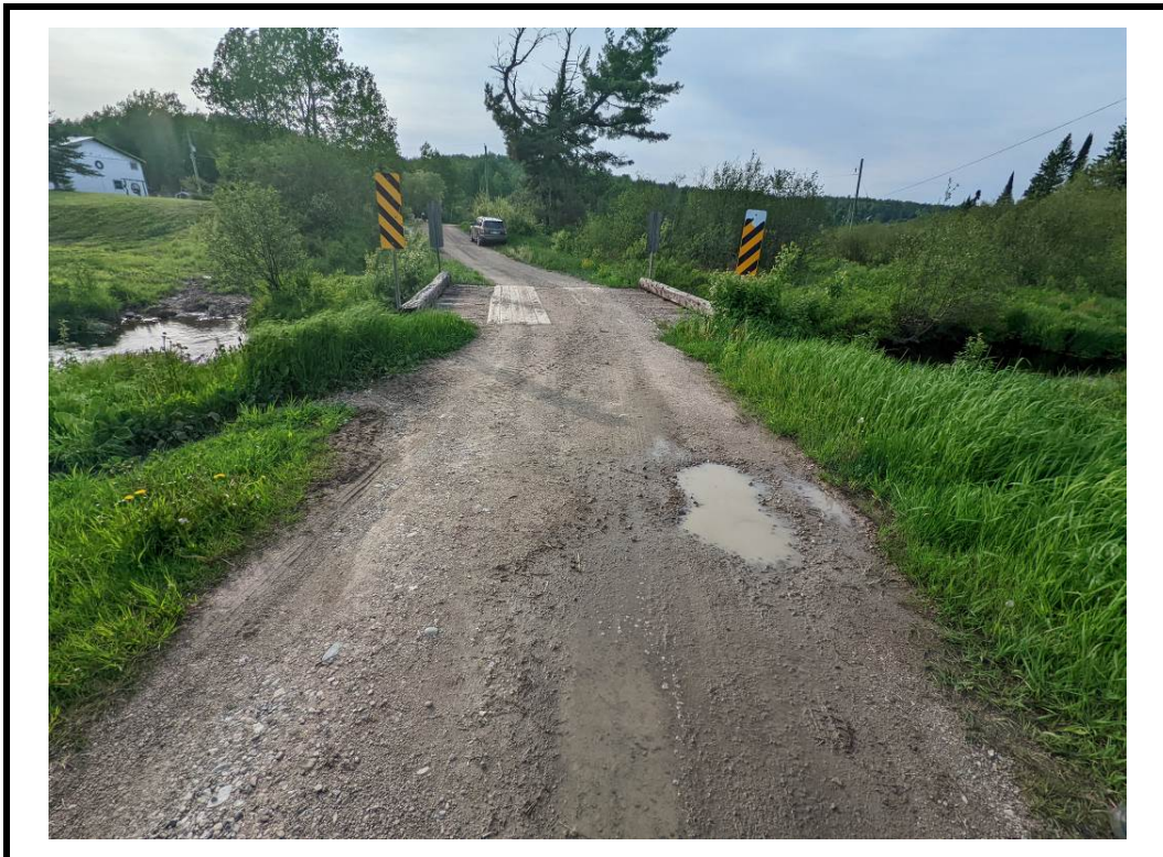
Photo 2 Structure from south approach
