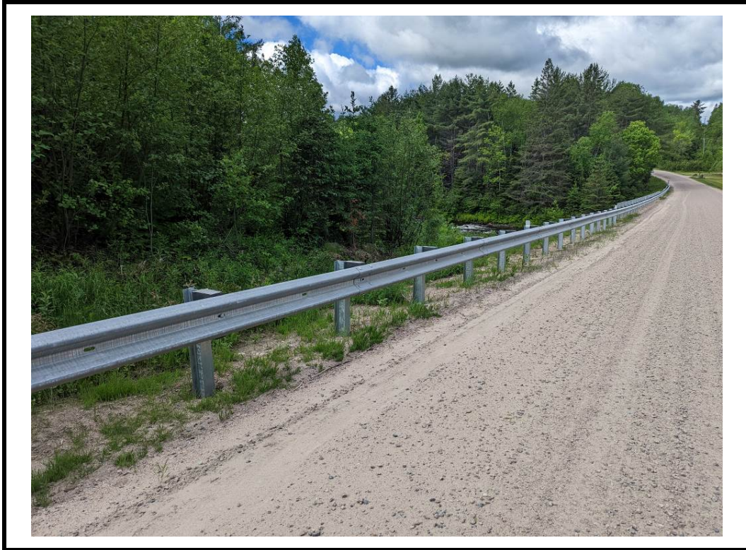
Photo 7 Typical approach barrier at southeast corner
