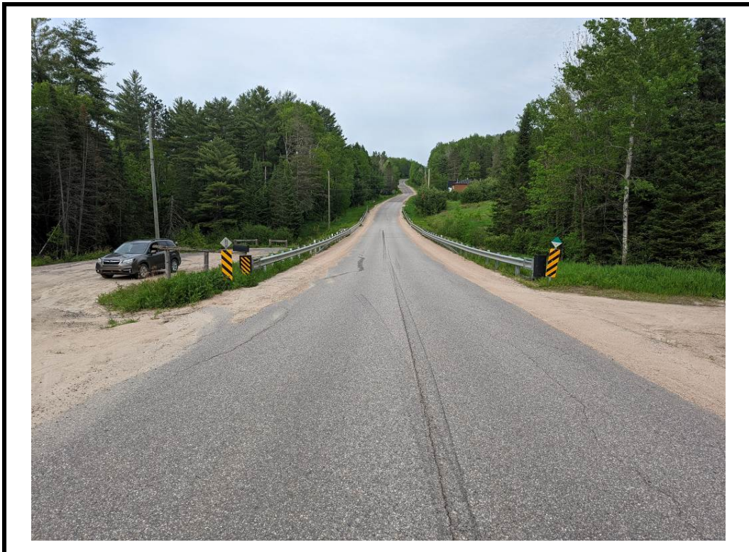
Photo 2 Structure from west approach
