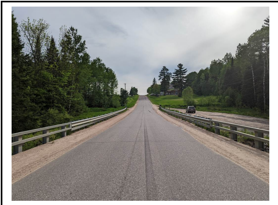
Photo 4 West approach from centre of structure
