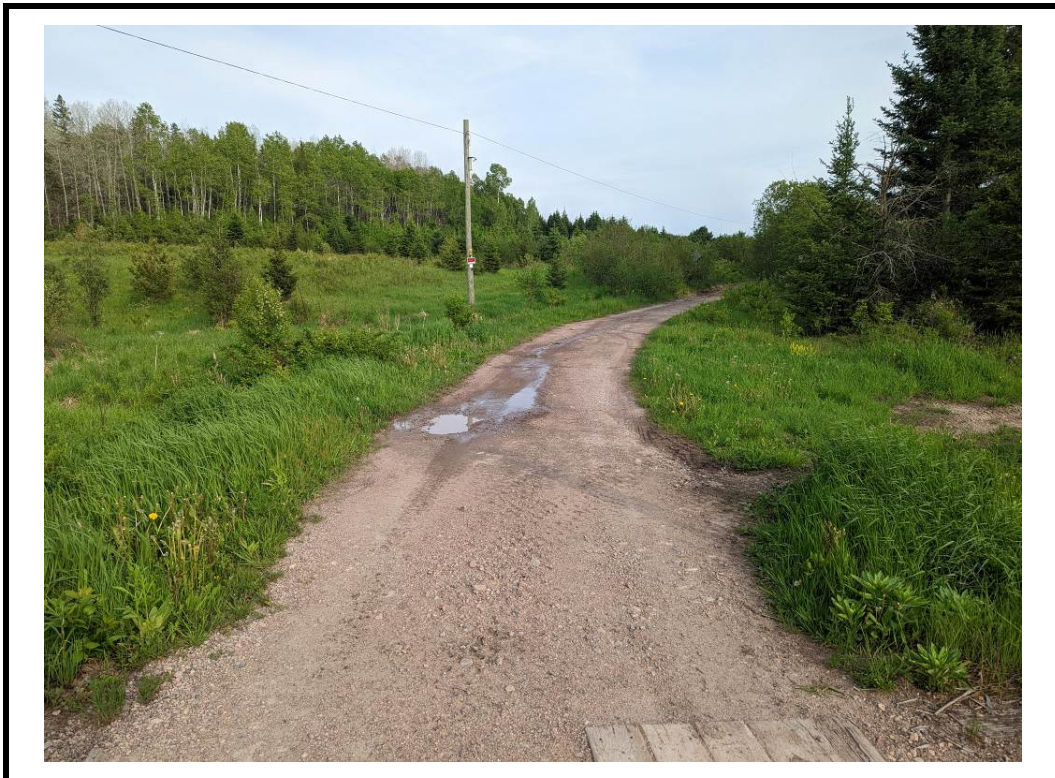
Photo 4 South approach from centre of structure
