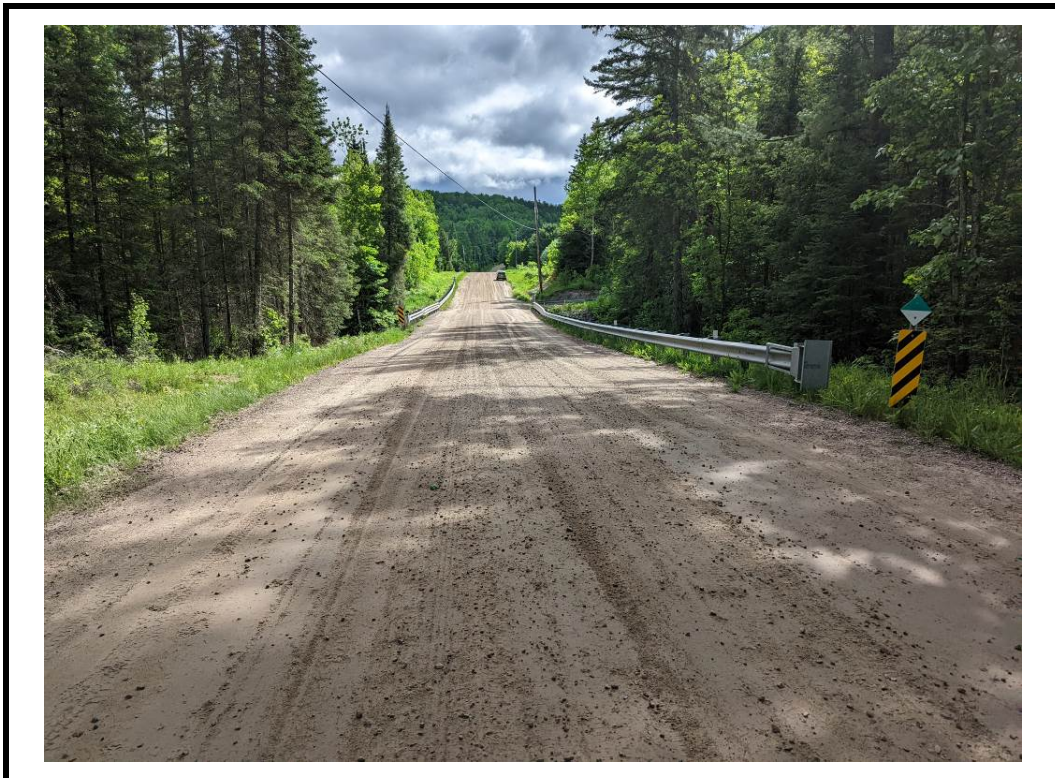
Photo 2 Structure from west approach
