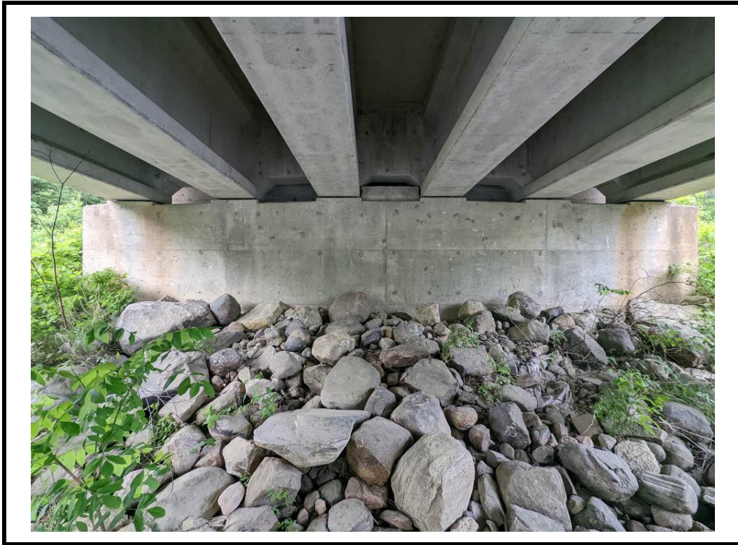
Photo 13 East abutment wall
