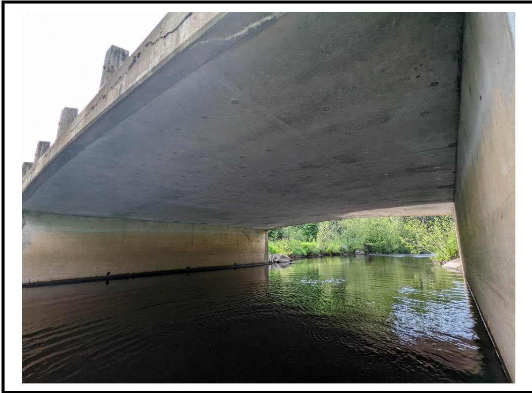
Photo 9 Underside of structure
