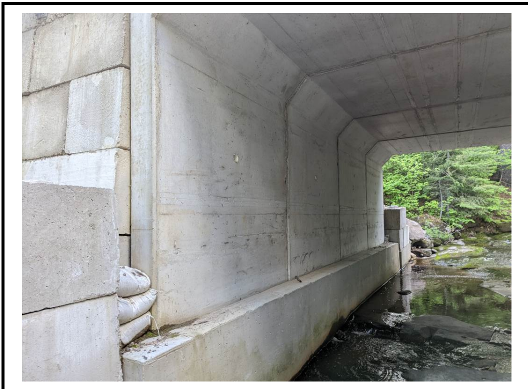
Photo 12 East abutment wall
