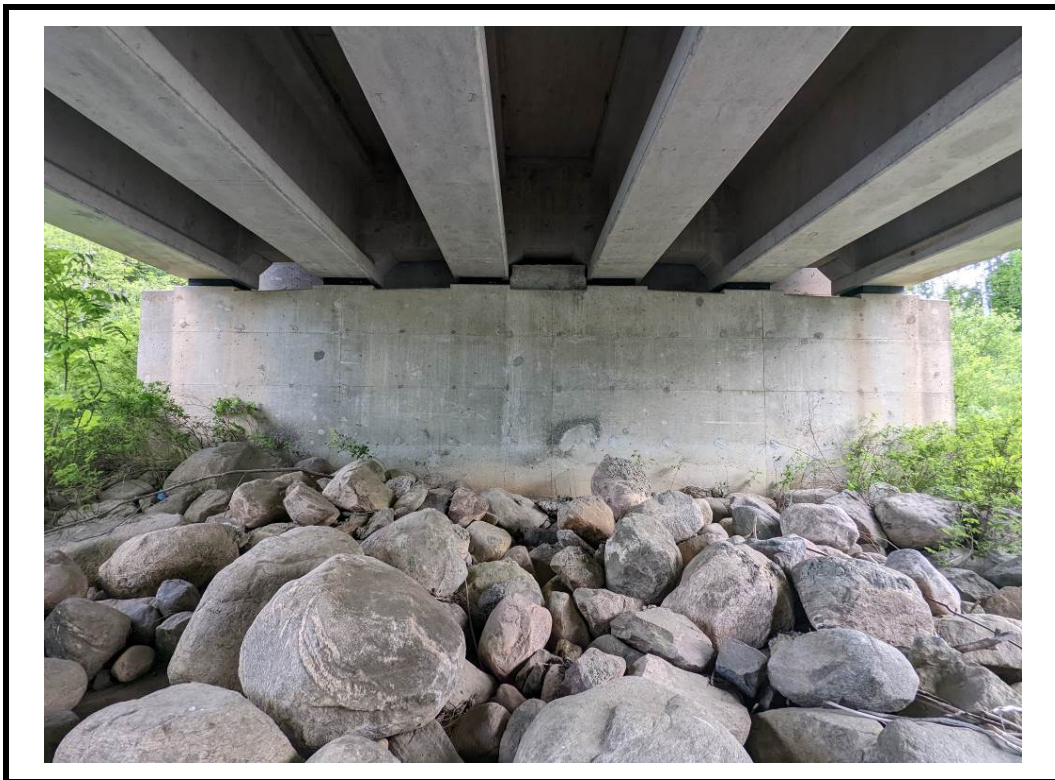
Photo 14 West abutment wall
