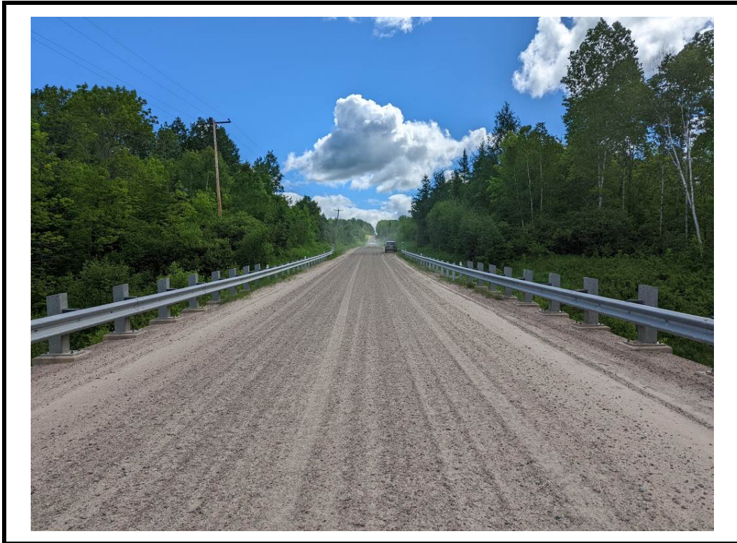
Photo 3 East approach from centre of structure
