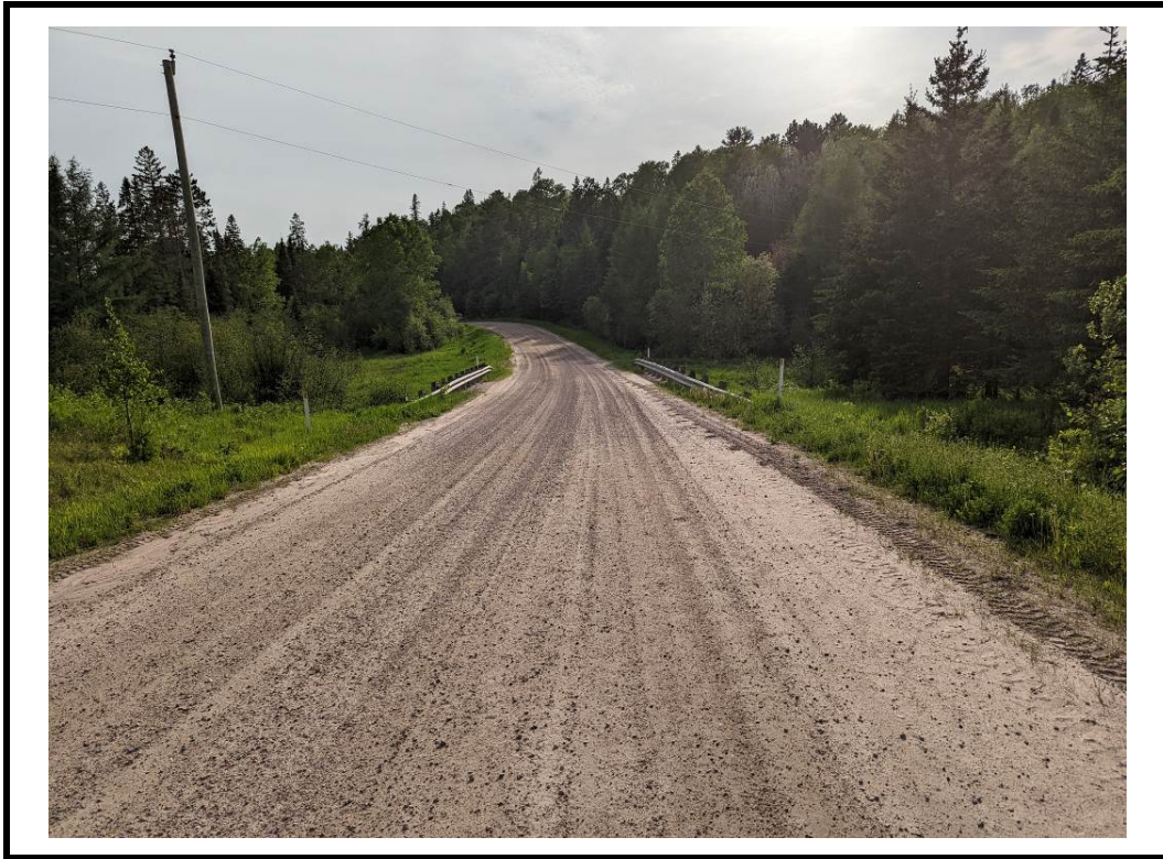
Photo 1 Structure from east approach
