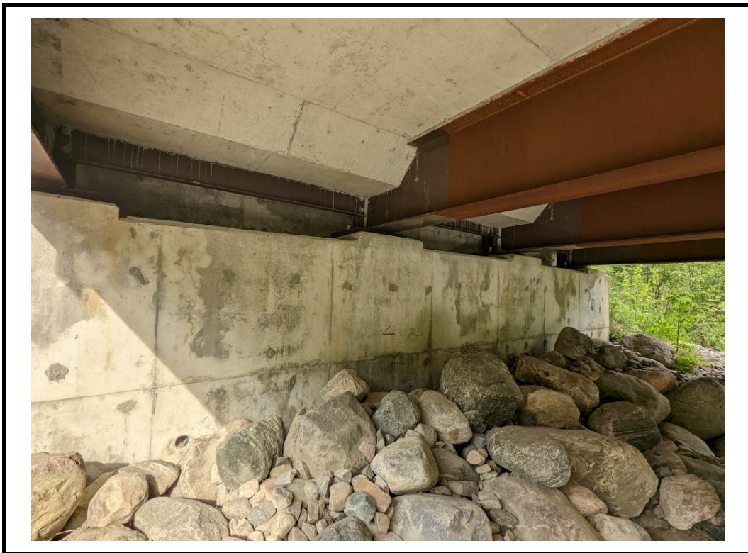
Photo 10 East abutment wall
