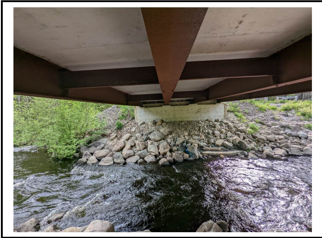
Photo 9 East underside of structure
