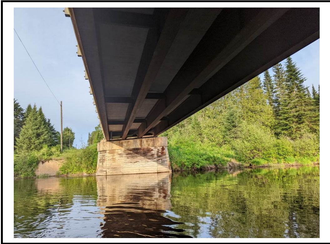
Photo 11 Middle span underside
