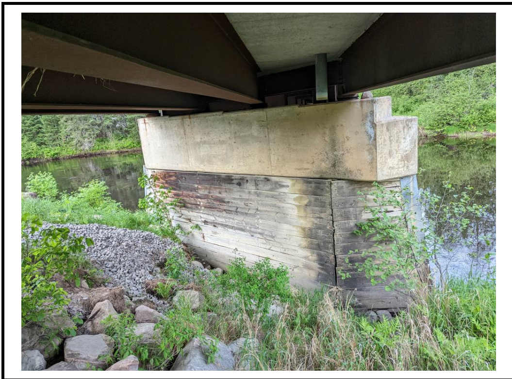
Photo 14 West pier and pier cap
