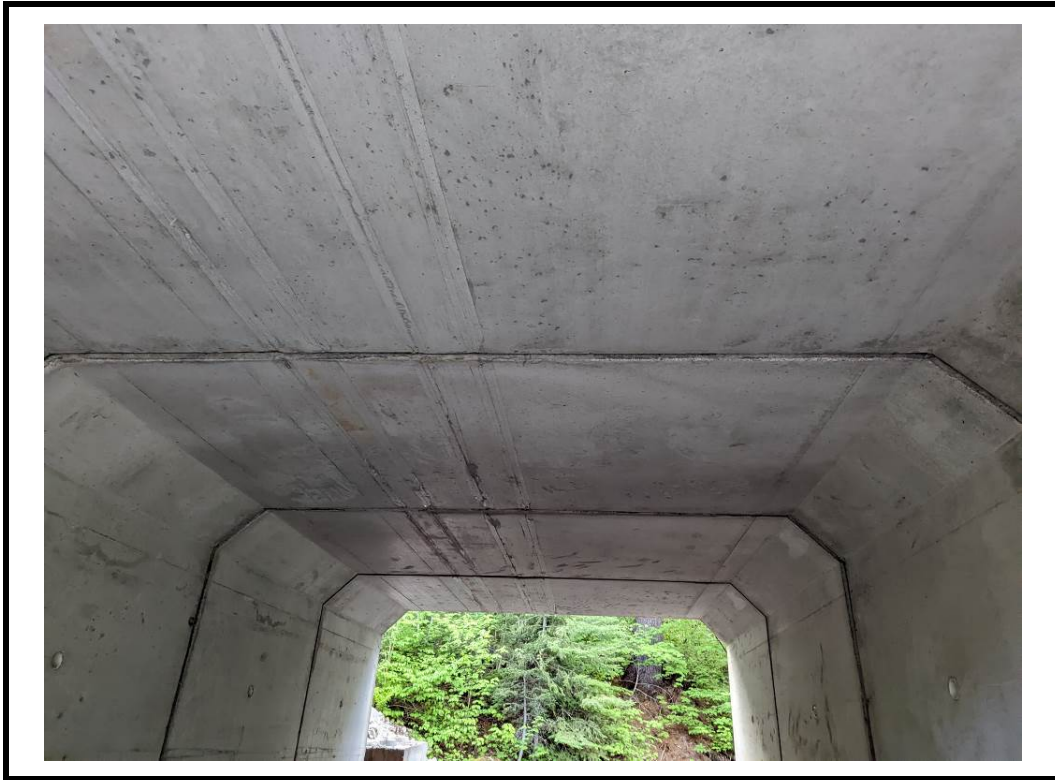
Photo 9 Culvert barrel soffit
