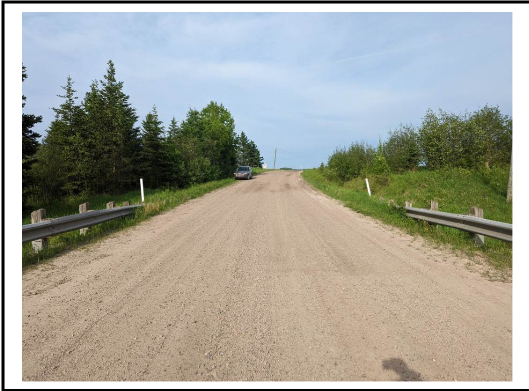
Photo 3 East approach from centre of structure
