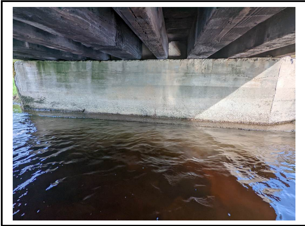
Photo 13 South abutment wall
