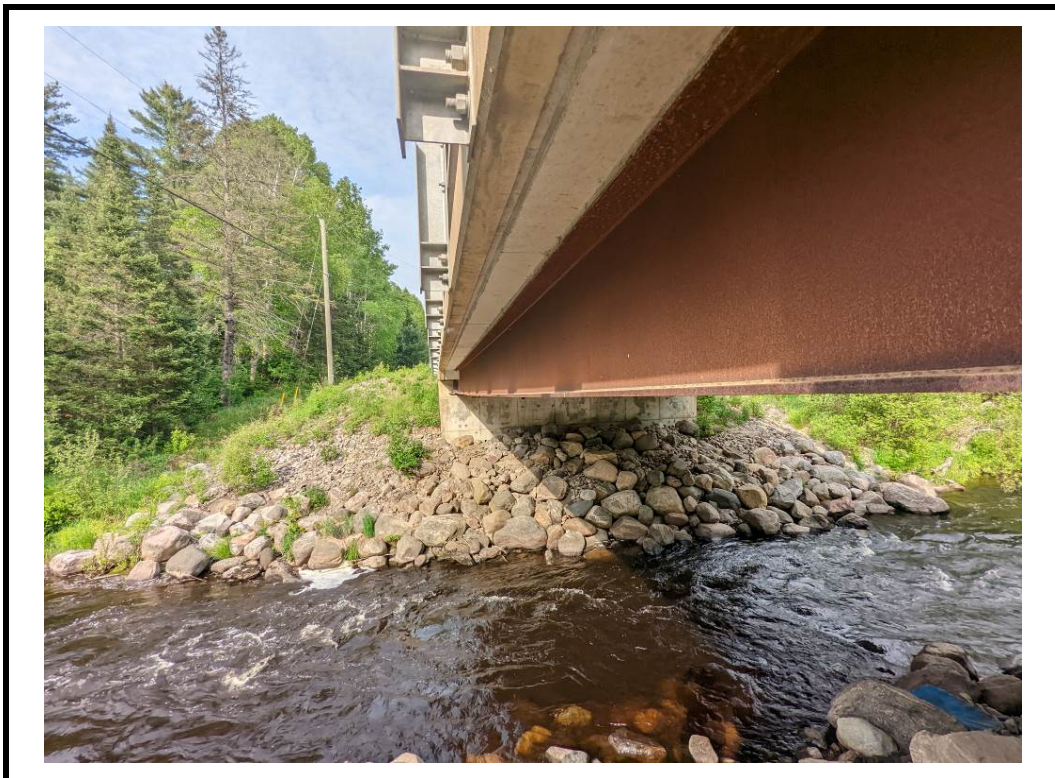
Photo 8 Typical end of steel girder at south side of structure
