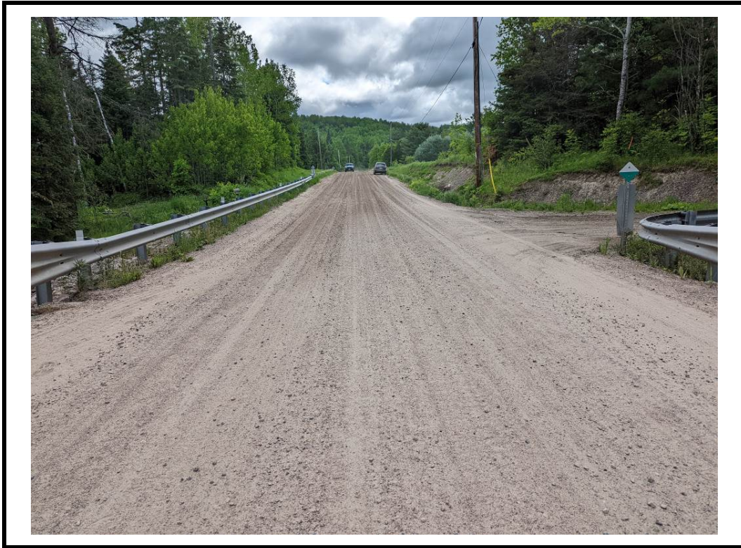
Photo 3 East approach from centre of structure
