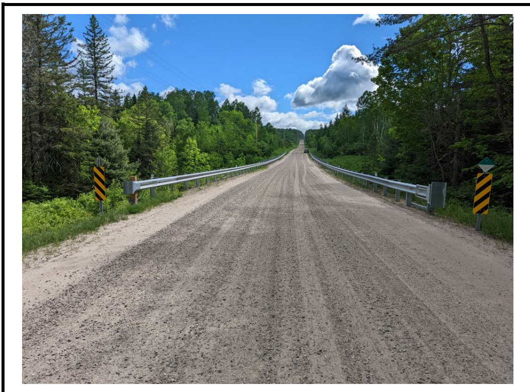
Photo 2 Structure from west approach
