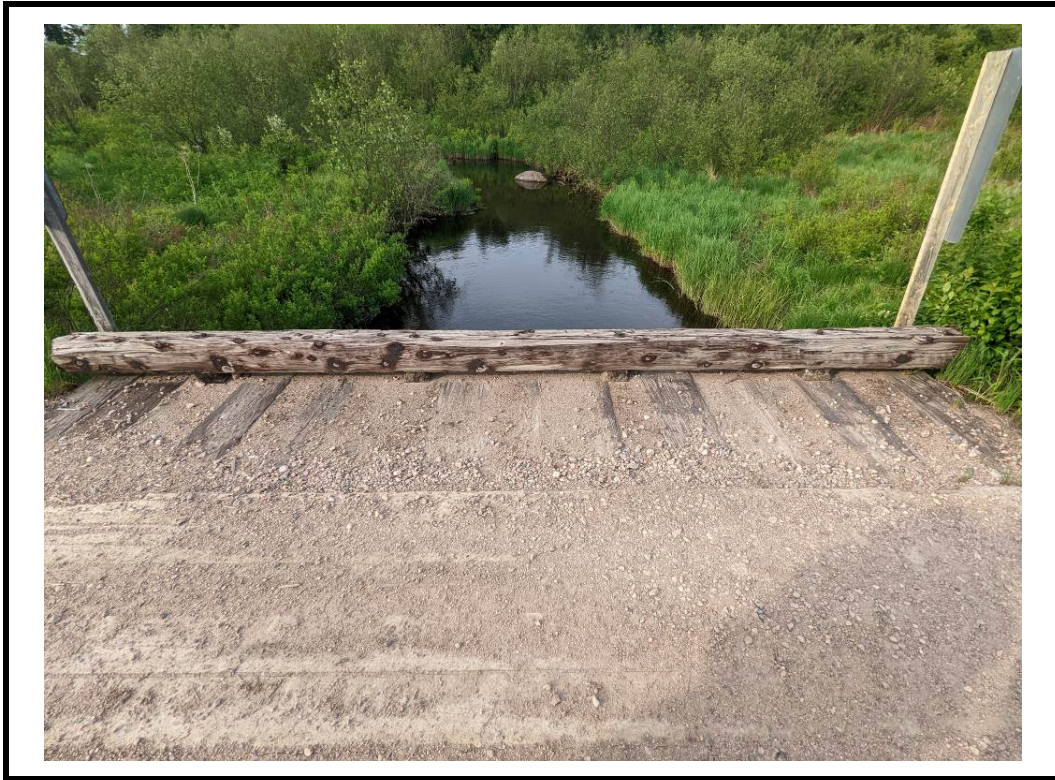
Photo 9 Deck wearing surface
