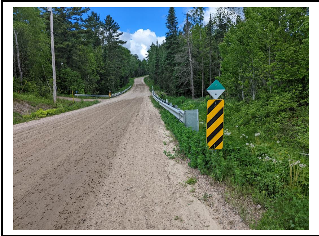
Photo 7 Northeast approach end treatment
