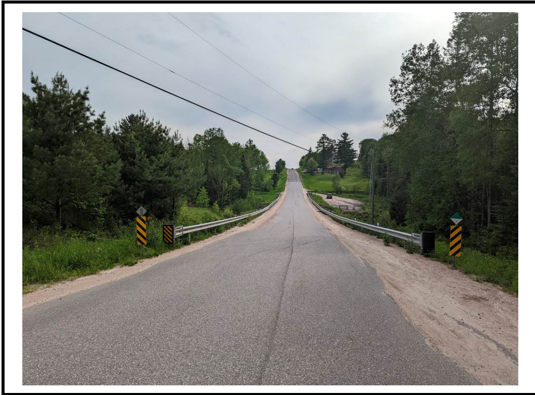
Photo 1 Structure from east approach
