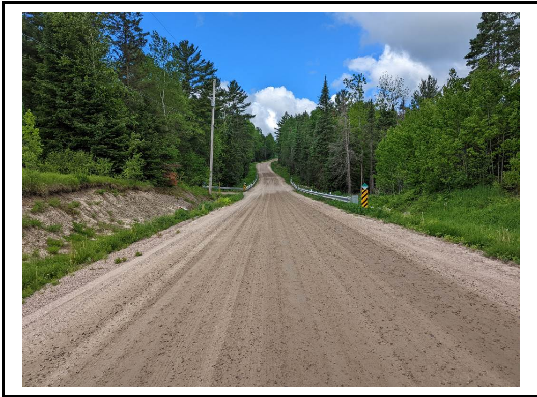
Photo 1 Structure from east approach
