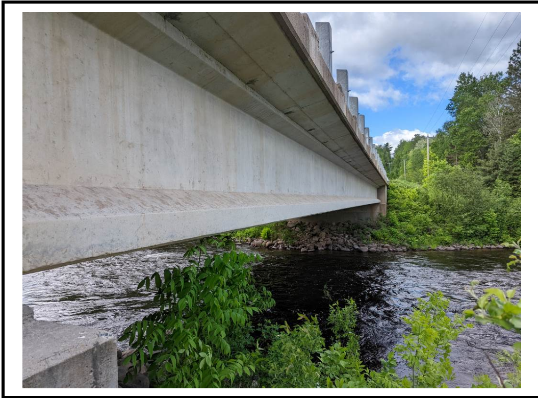
Photo 17 Typical view of exterior girder at north side
