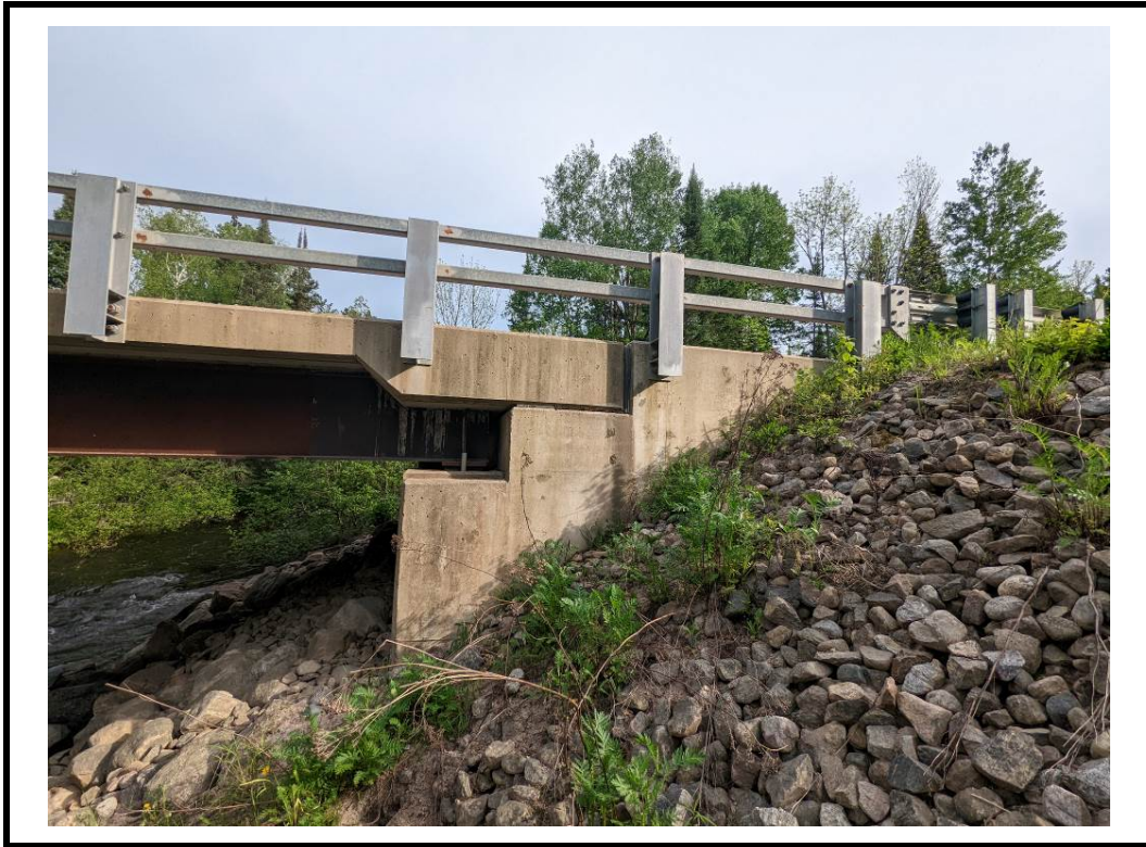
Photo 13 Typical southeast wingwall
