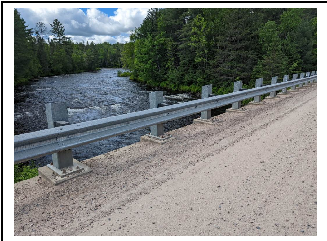
Photo 10 Typical deck barrier at south side of structure
