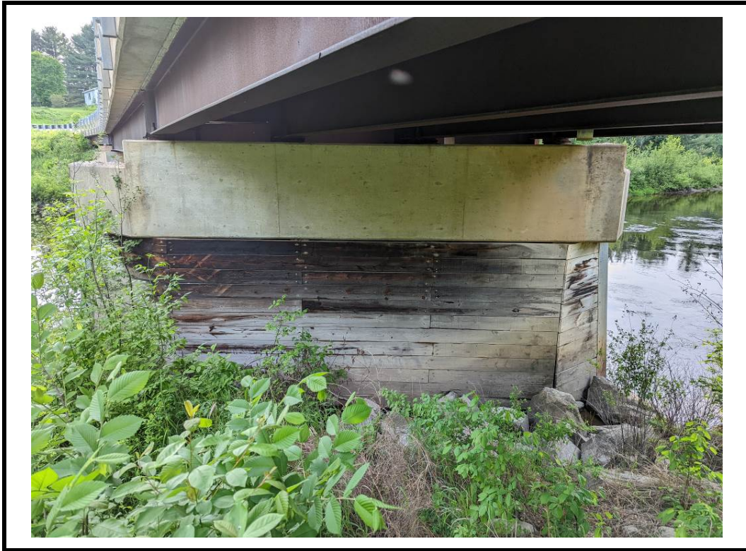
Photo 13 East pier and pier cap
