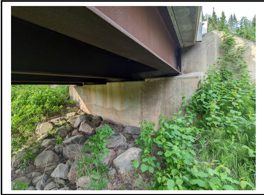
Photo 15 East abutment wall
